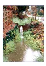
LID stormwater designs mimic natural drainage processes by using stormwater site design and best management practices that retain vegetation, limit impervious surfaces, and infiltrate runoff onsite.
