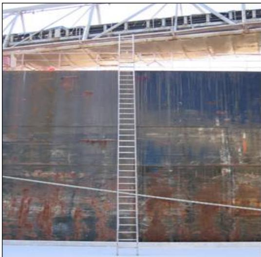
*This is a 10-meter [nearly vertical] climb and the ladder is not safely secured at the top or bottom.*
