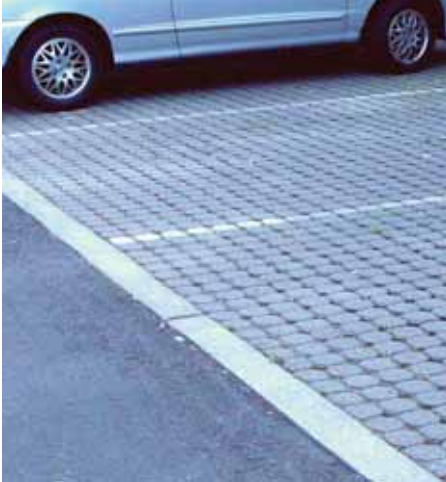
Permeable pavement like this provides a hard, drivable surface, but it also lets some stormwater soak back into the ground.
