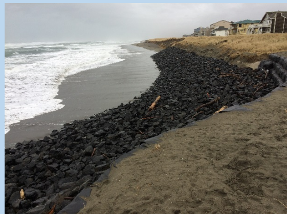
USACE Emergency Rock Revetment, Jan. 2016
