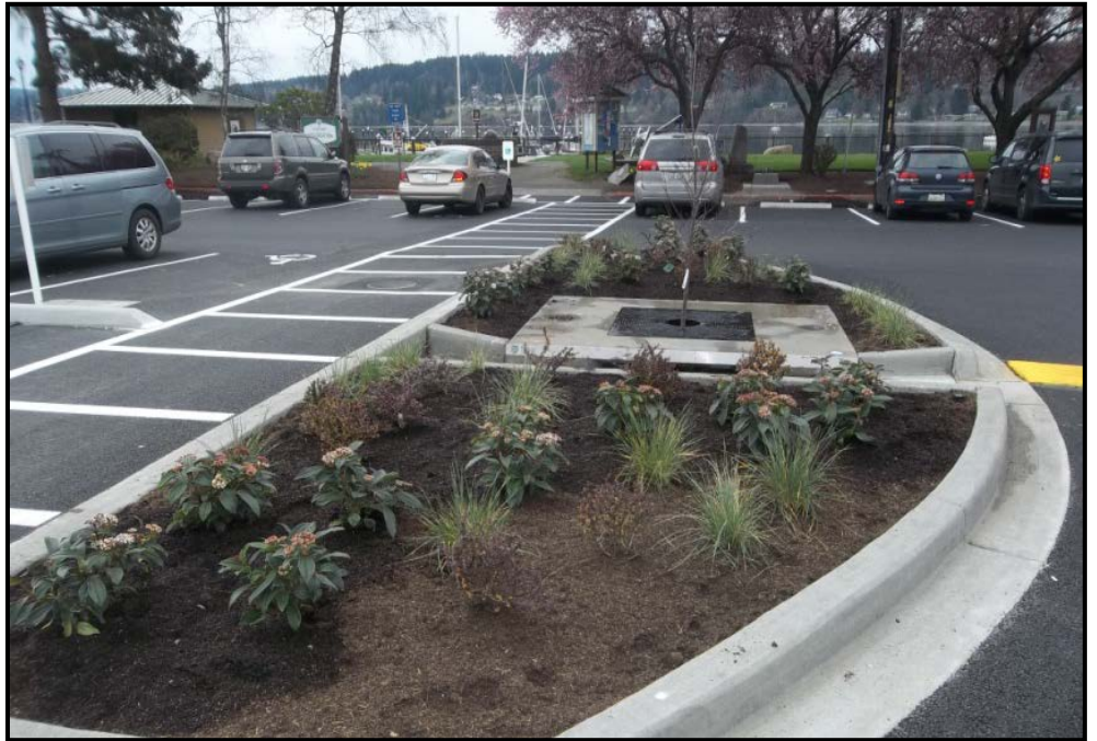
Anderson Parkway “after”. Looking at parking lot near Liberty Bay. Picture shows bioretention cells and the top of a Filterra unit in the middle. These clean stormwater from parking lot and add attractive plantings.
