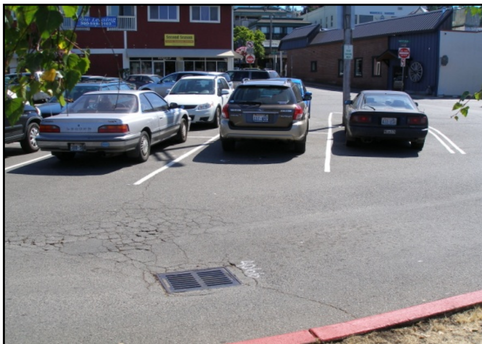
Anderson Parkway "before." Looking at parking lot from the bay side. Stormwater goes untreated into storm drain to Liberty Bay.
