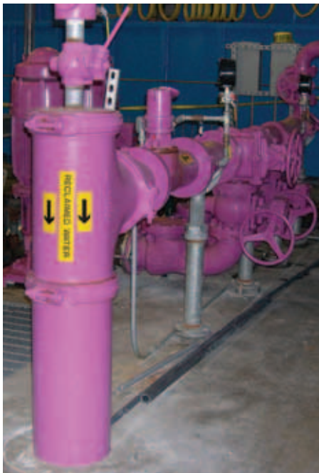
Purple pipes at Medical Lake treatment facility carry water to Medical Lake and Deep Creek.
