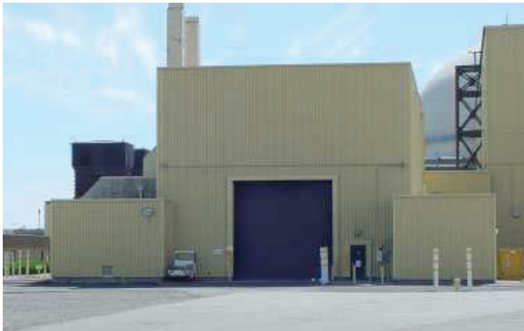
Fuel Storage Facility (FSF) Building 403
