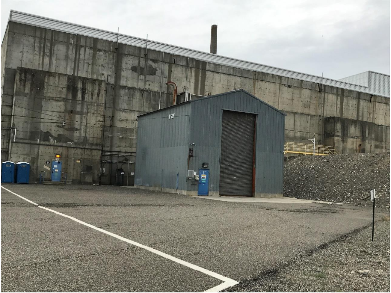
1 Figure H-2 T Plant 277-T Building Exterior (Looking Southeast) (May 2017)
