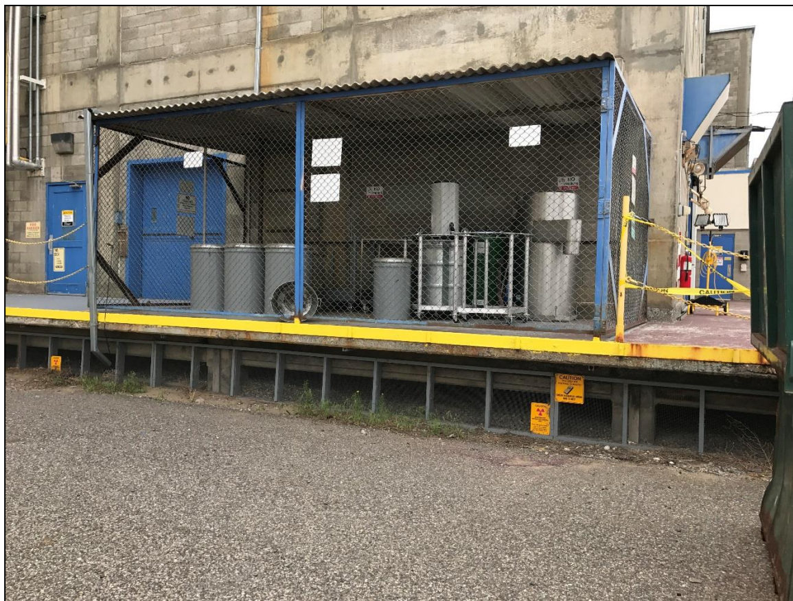
1 Figure H-2 T Plant 271-T Cage Outdoor Container Storage Area (May 2017)
