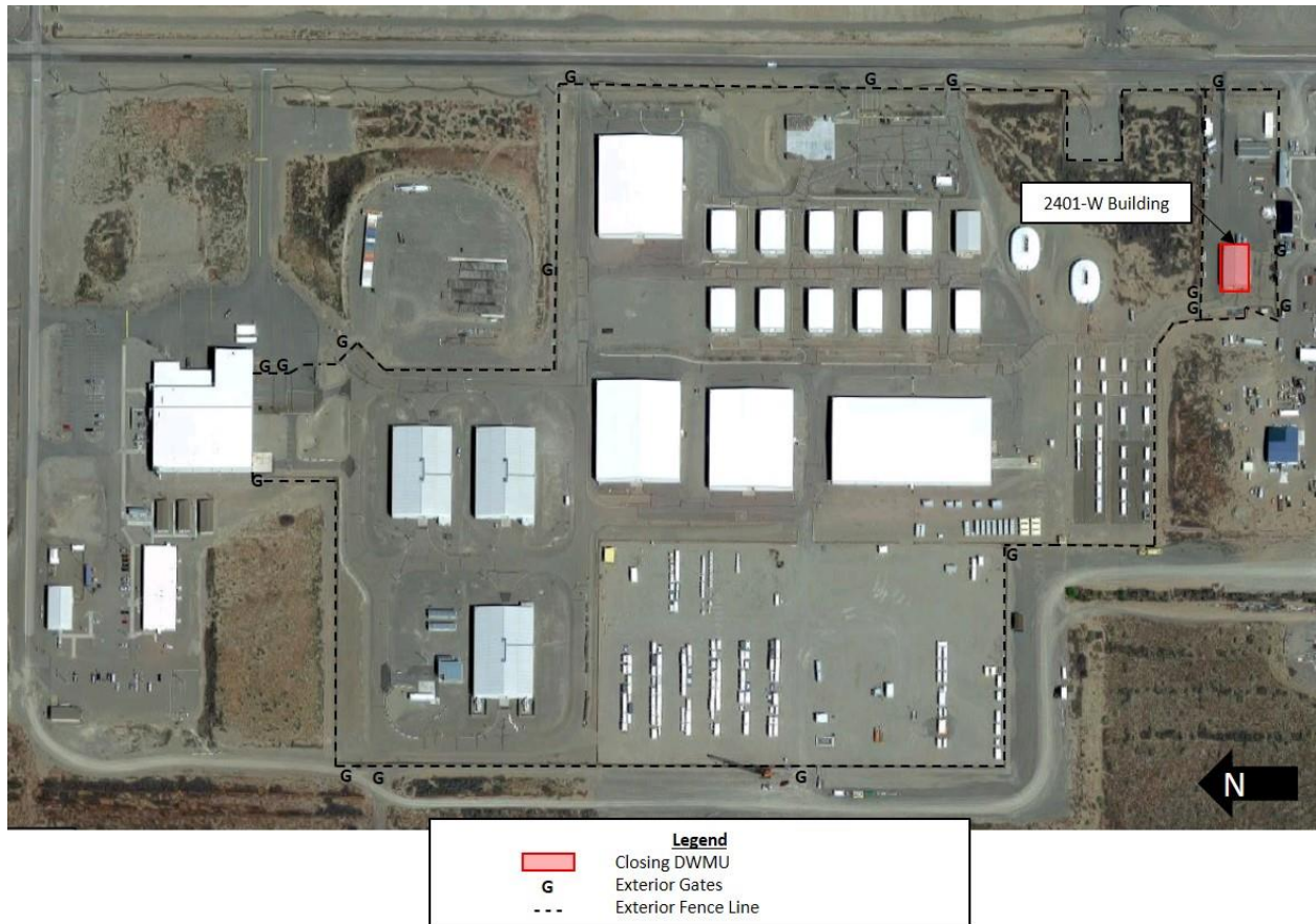
1 Figure H-1 Central Waste Complex-Waste Receiving and Processing Complex Overview, 2 2401-W Building Dangerous Waste Management Unit (Month Unknown, 2017) 3
