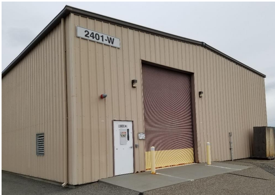
Figure H-3 2401-W Building (East) (February 2018)
