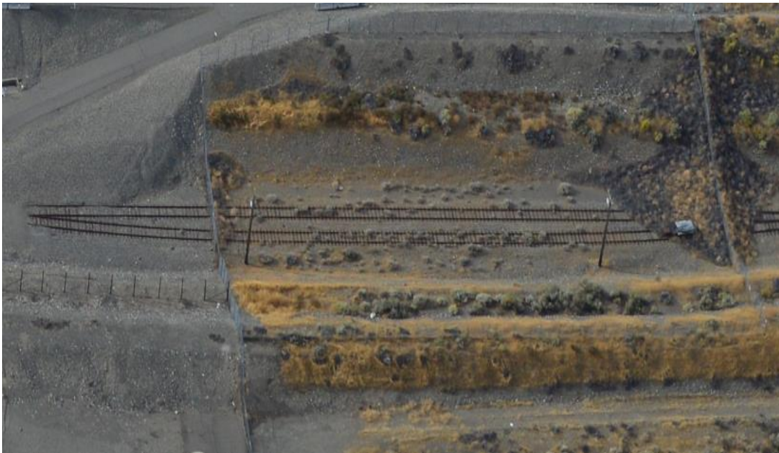
2 Figure H-3 Overhead View of 221-T Railroad Cut from Southwest (October 2017)
