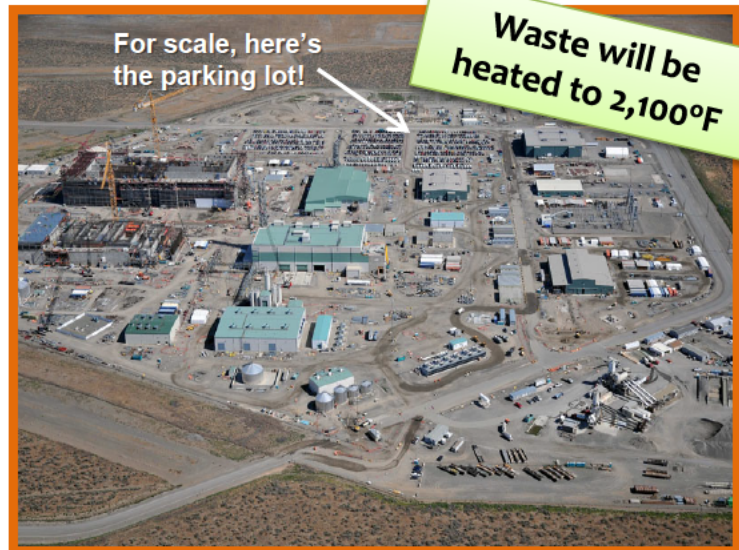
Aerial view of construction, July 2011
