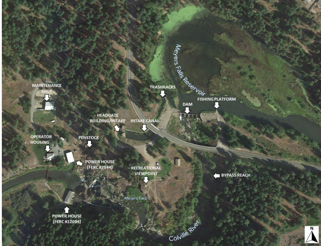
Figure 1. Meyers Falls Hydroelectric Project Facility Layout
