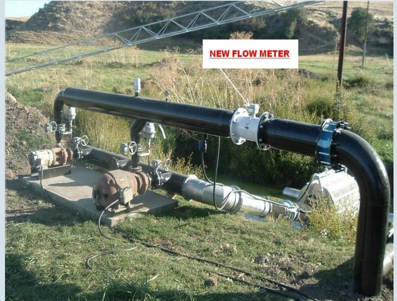
Flow Meter and River Fish Screen at irrigation diversion
