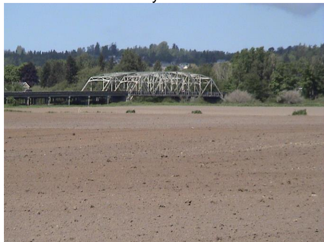
Looking South to Interstate 5 Bridge
