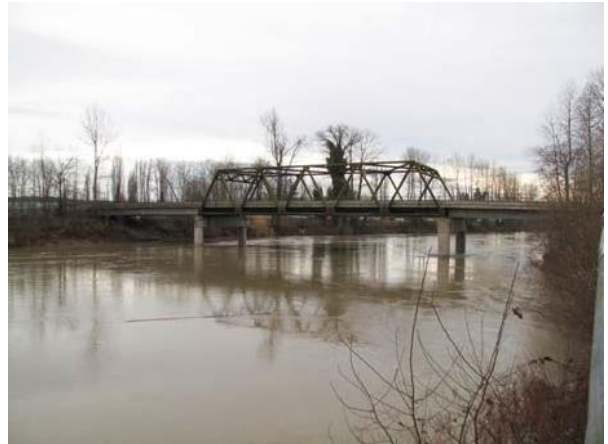
Avenue D bridge over Snohomish River
