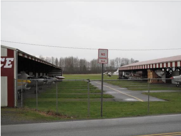
Harvey Field airport facilities in mapped floodplain south of river
