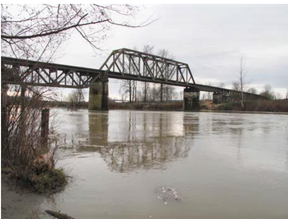
Railroad trestle bridge
