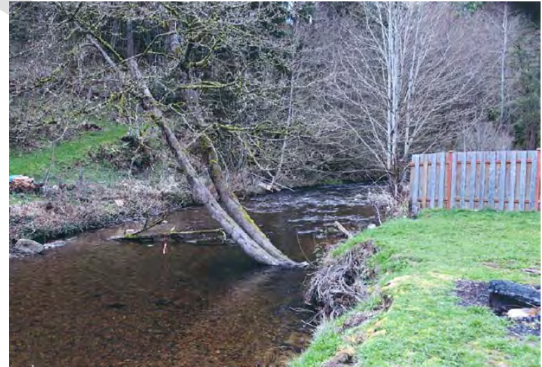
Photo 8: Reach 1c: View downstream showing bank erosion downstream of the incised reach. Photo J from Wilkeson's first draft Inventory and Characterization
