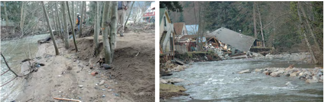
Photo 9: Photo 9a on left shows flood deposits on channel left at head of channel migration section. Photo 9b on right shows older aggradation as bars on channel right as well as damage caused by channel migration.
