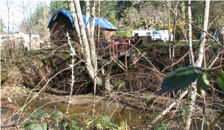
Photo 7: Reach 1c: Aggradation and bank failure occurring in incised channel.
