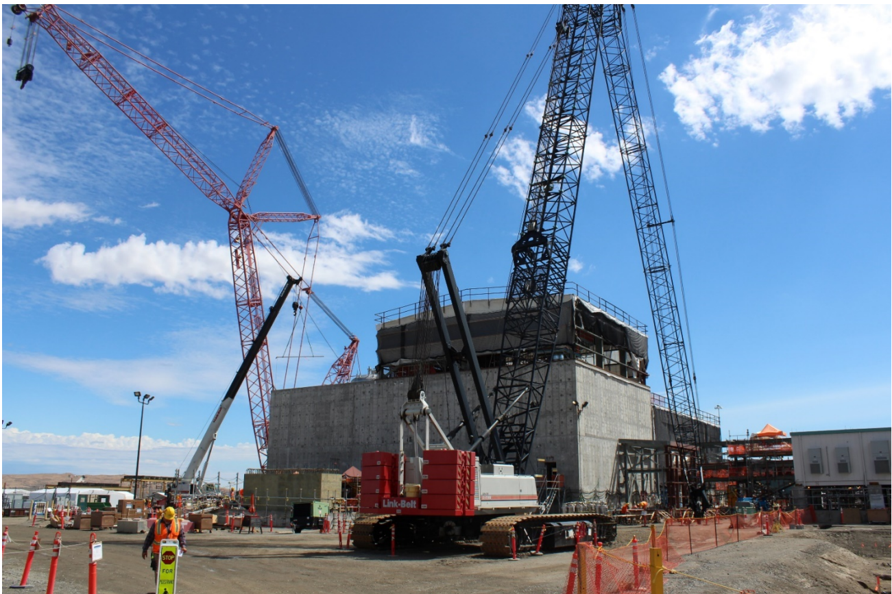
Figure 1 Effluent Management Facility
