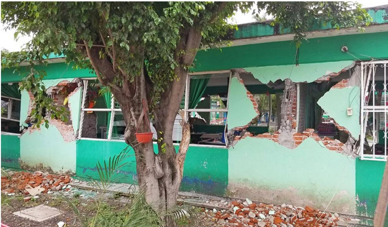
**Figure 9.** Structural earthquake damage to a primary school in central Mexico from the 2017 M7.1 Central Mexico Earthquake (Photo by Reid Middleton, Inc.).
